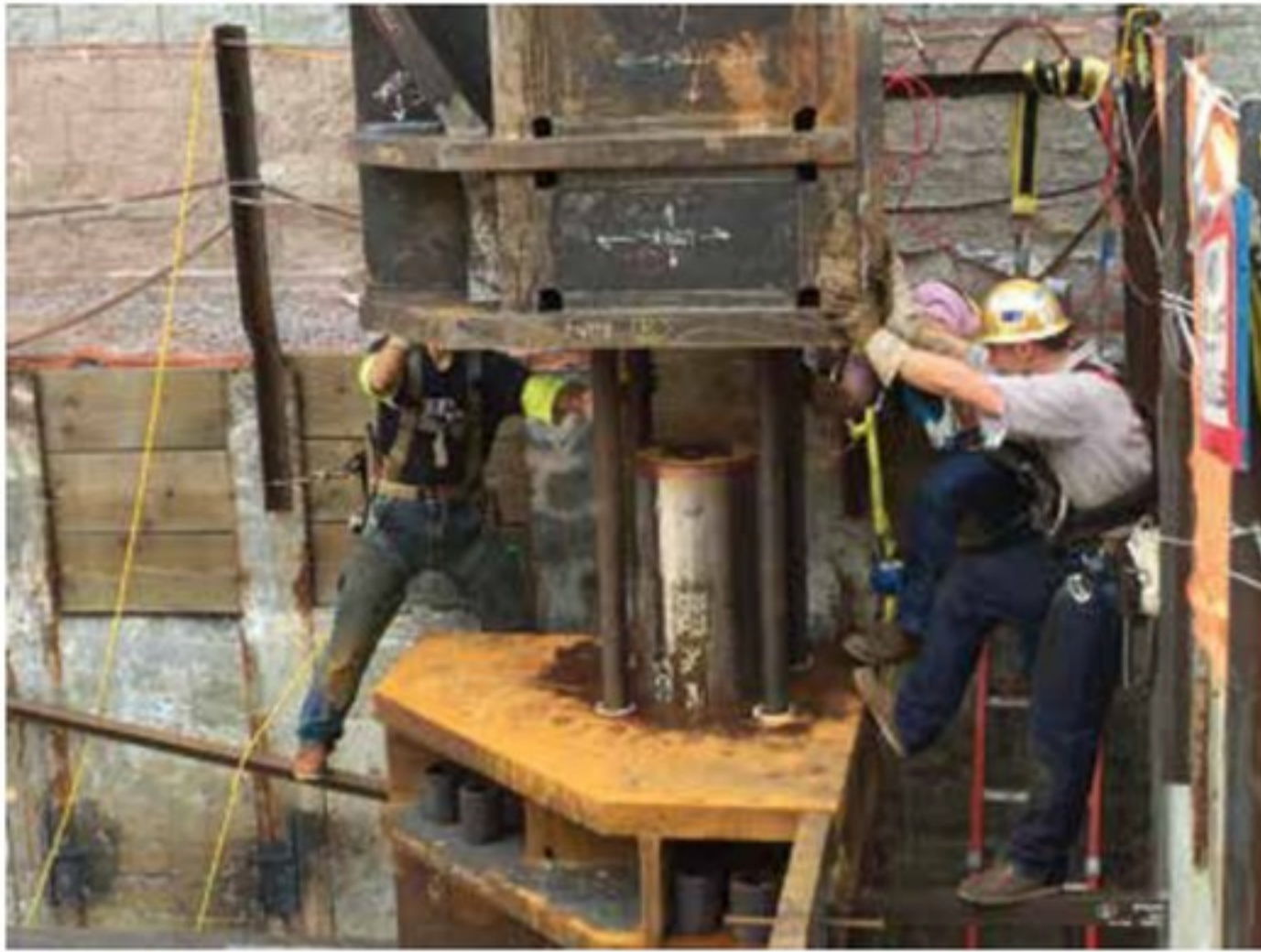
Figure 5. Construction workers are lowering the mega-column base over the shear key.
