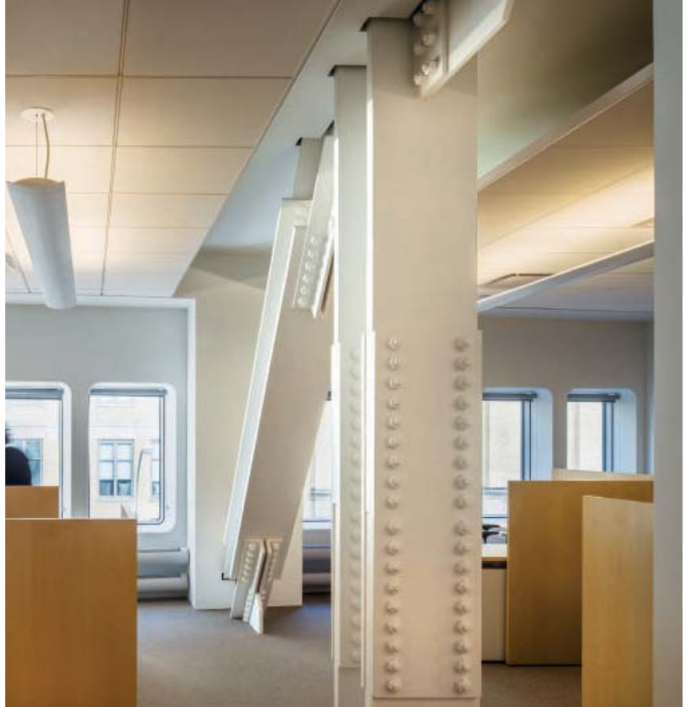
The structural supports for the building's large cantilevers remain visible as points of interest within the museum.
